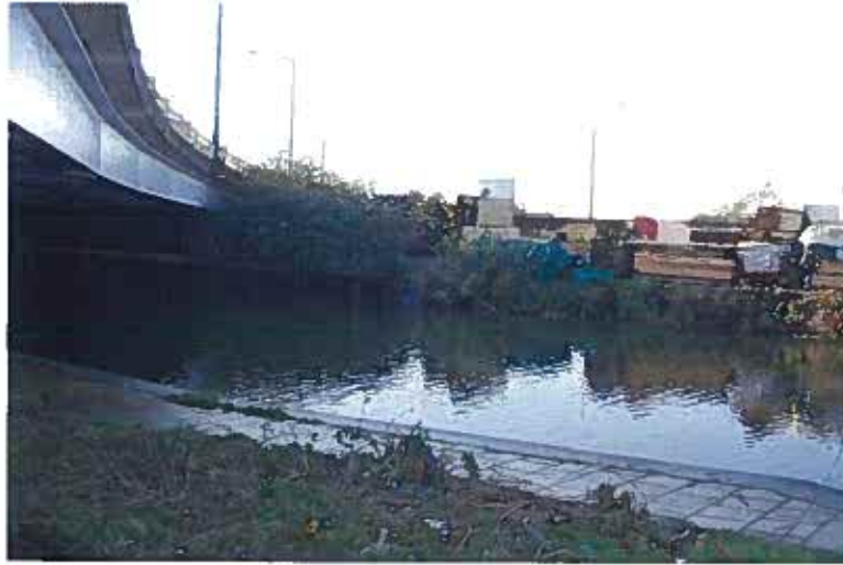
Figure 2 Looking towards the west bank of the river Lee opposite the footpath sign to Angel Road station above
