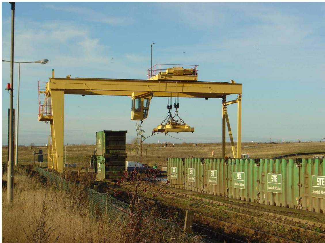
Residual waste is transported to landfill by rail.
