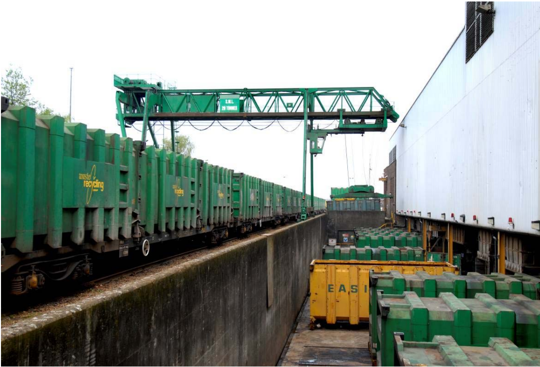
Residual waste is loaded into containers at the Hendon Rail Transfer Station.
