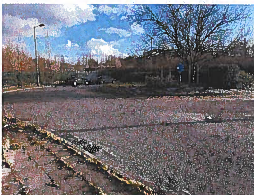
Orion Road Roundabout
