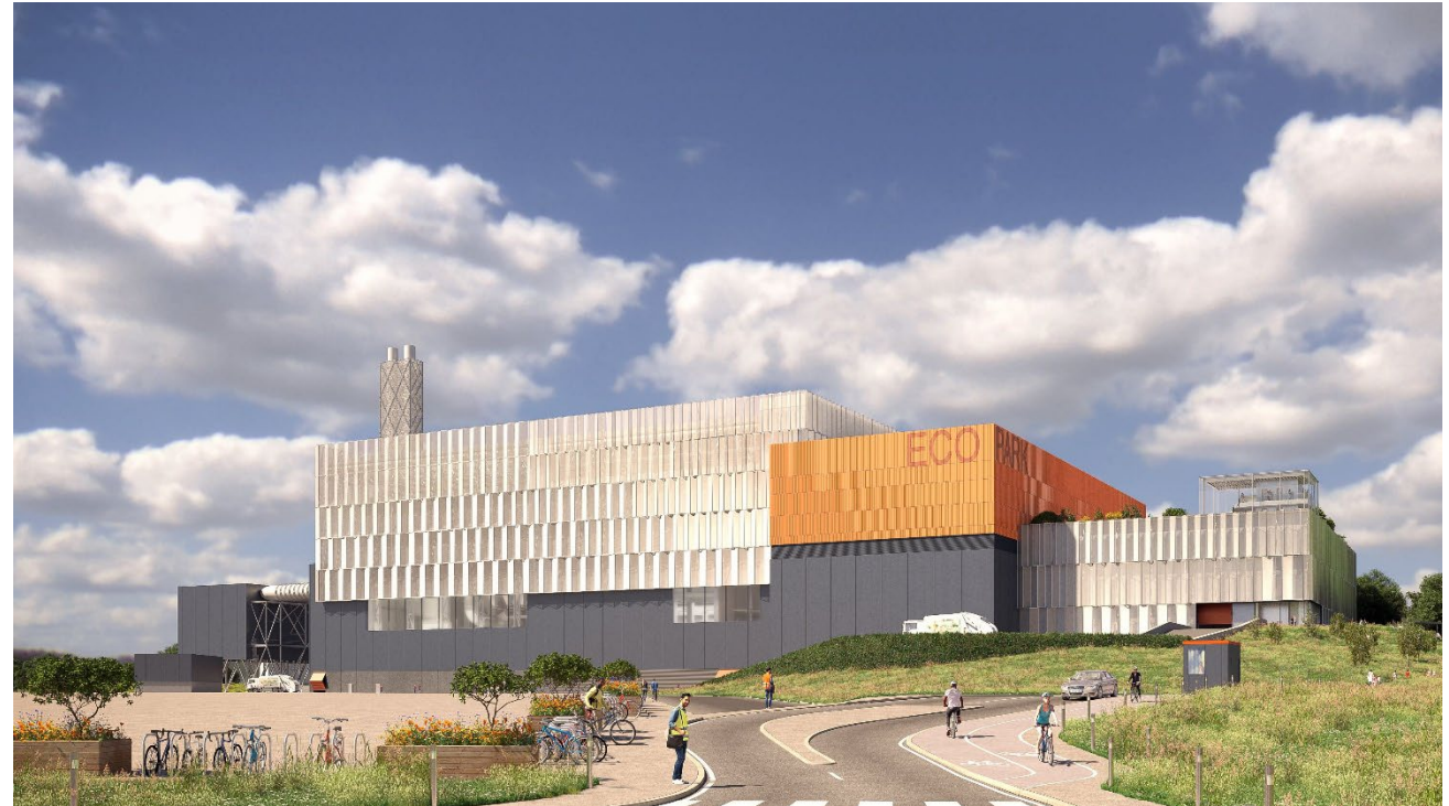
The Energy Recovery Facility
