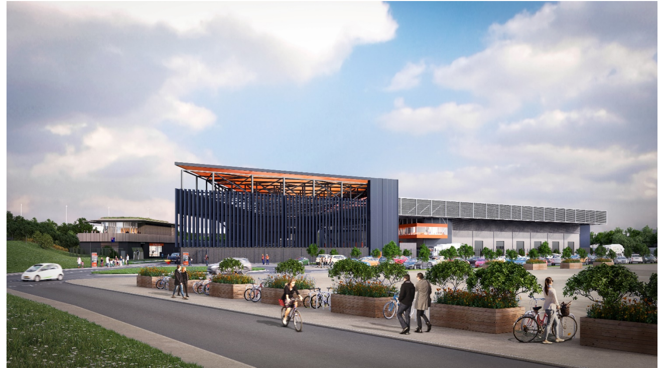
The Resource Recovery Facility
