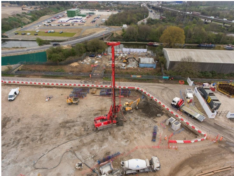
Image 1: Piling works being undertaken on EcoPark South, North London Heat and Power Project
