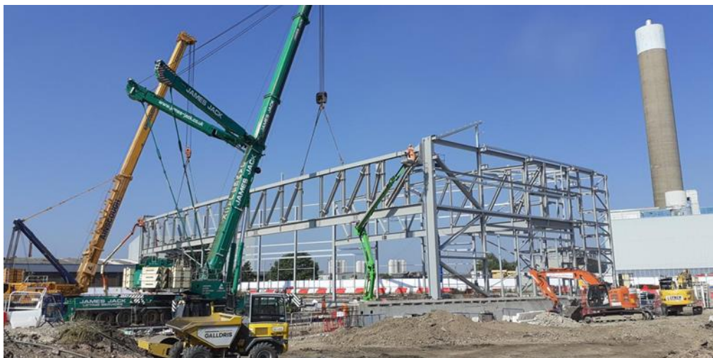
Figure 2 RRF steelwork construction site progress
