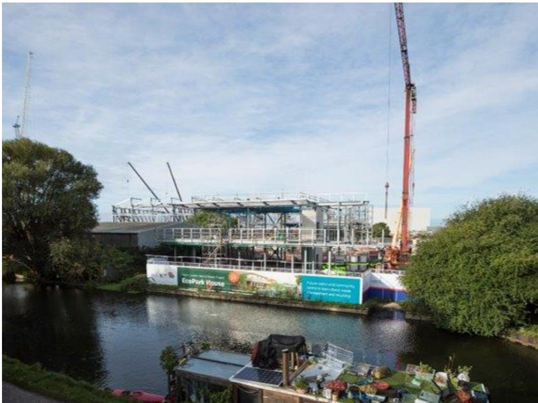
Figure 3 EcoPark House under construction
