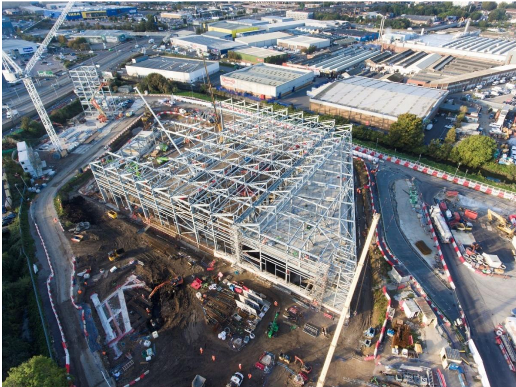
Figure 2 RRF Steelwork being erected
