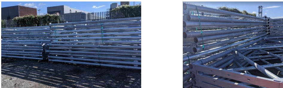
Figure 5 Steel truss frames stored on site
