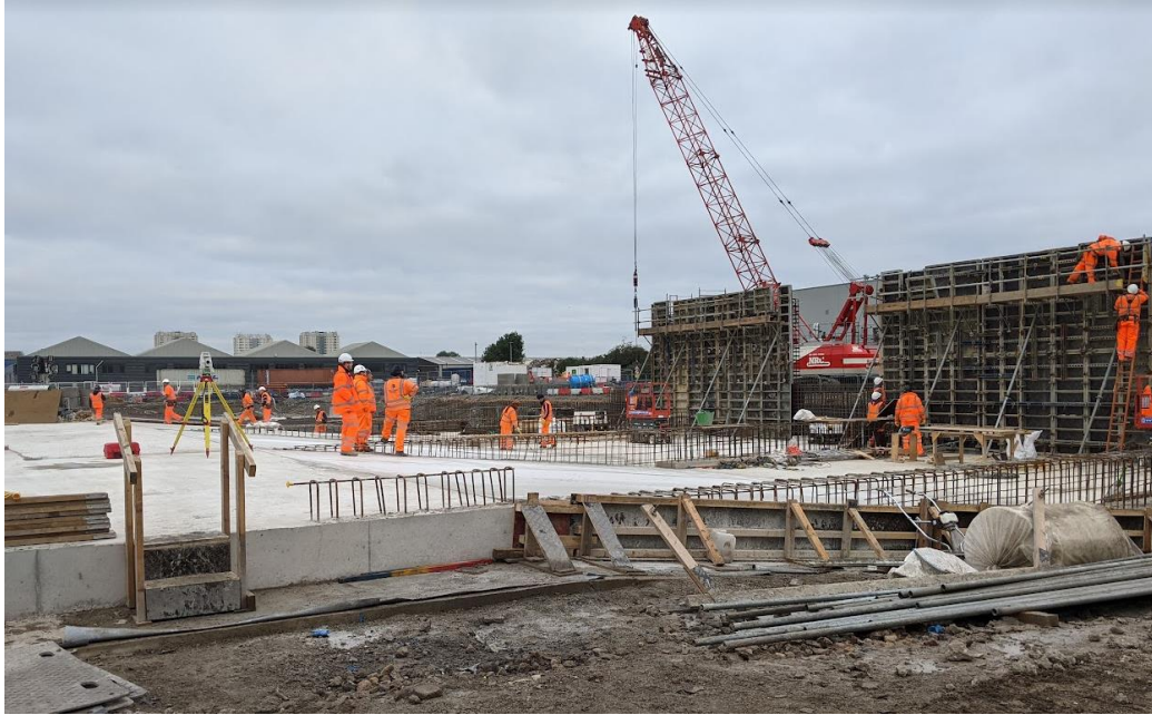
Figure 4 Construction of floor slab and walls
