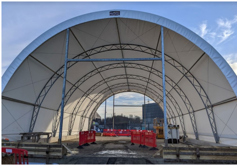
Figure 8: TBWRF workshop building
