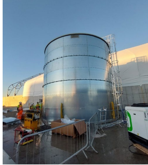
Figure 7: Fire water tank
