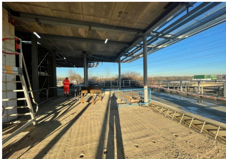
Figure 4 Progress on Eco Park House F01 – Membrane, Upstands & Blockwork
