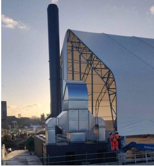
Figure 6: Odour plant installation
