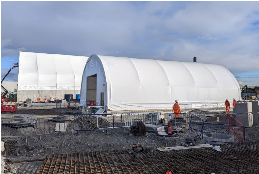
Figure 8 Workshop Building in the foreground
