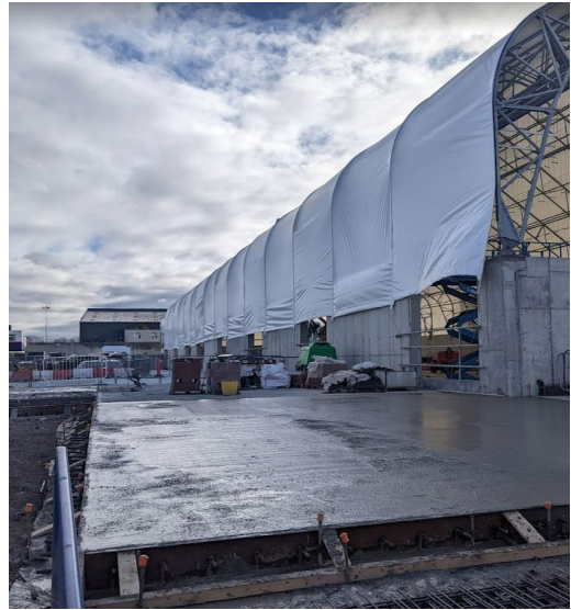
Figure 7 Roads Under Construction
