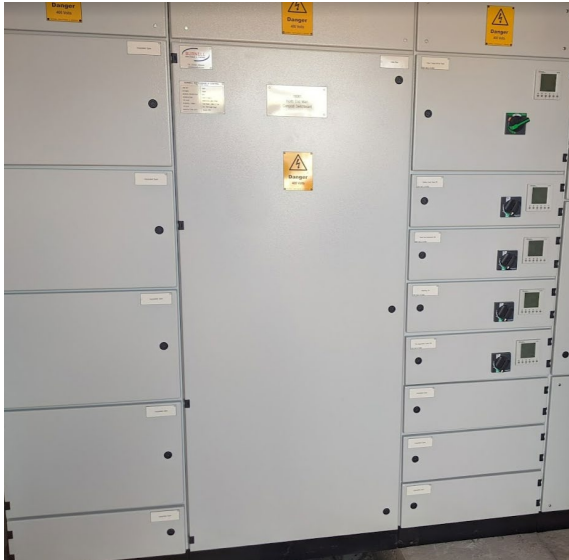
Figure 6 New Electrical Switchgear
