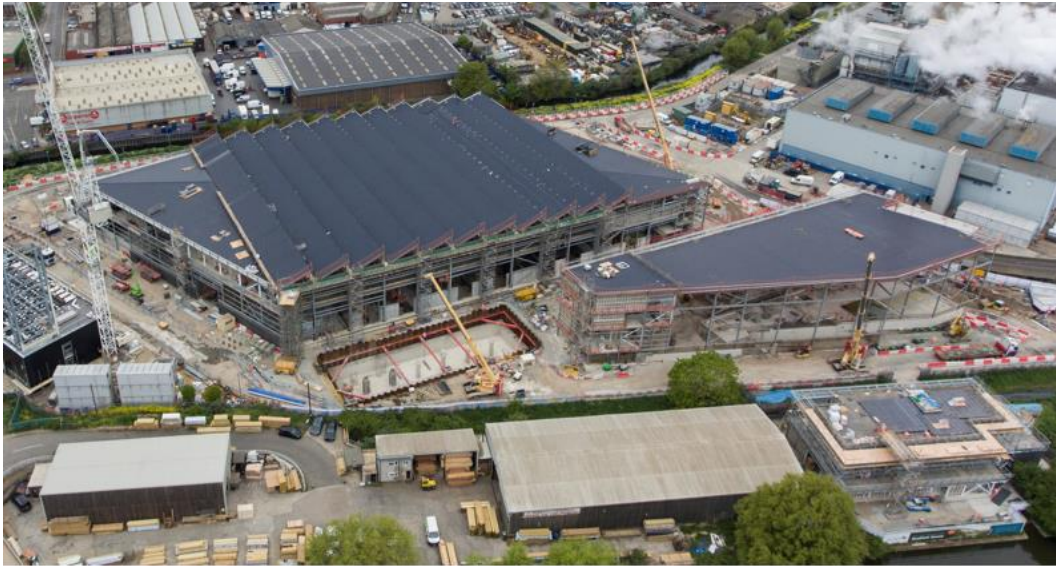
Aerial view of the RRF and RRC under construction with EcoPark House in the right foreground
