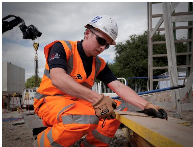
One of our many apprentices on site
