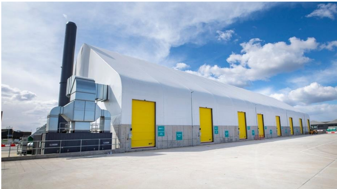
External view of the completed Temporary Bulky Waste Recycling Facility
