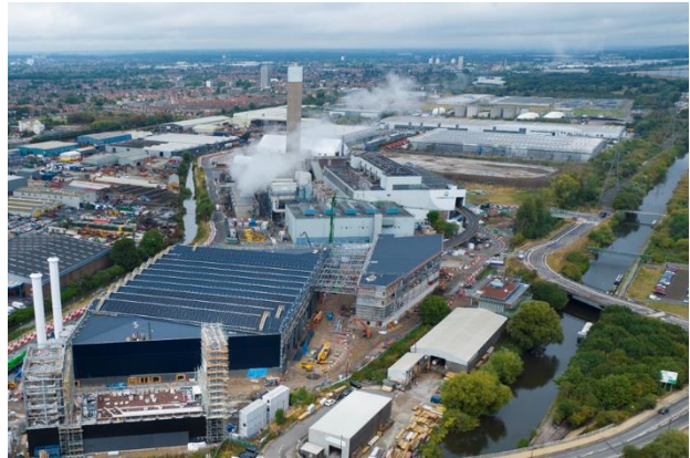
An aerial view including the odour control chimneys
