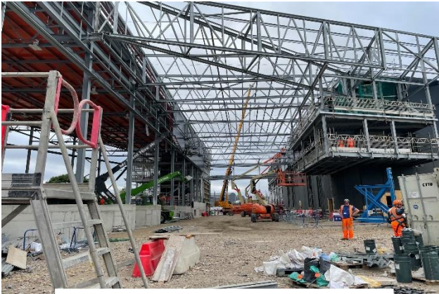
Steel work canopy link between the RFPF and RRC
