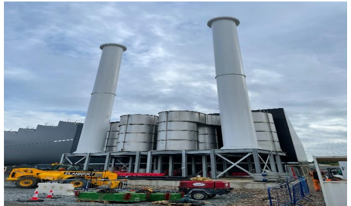
RRF showing the odour control stacks
