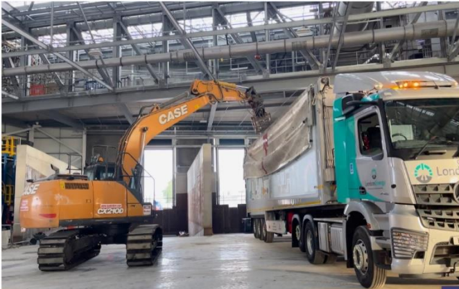
LEL Trialling Loading Operations on Tipping Apron
