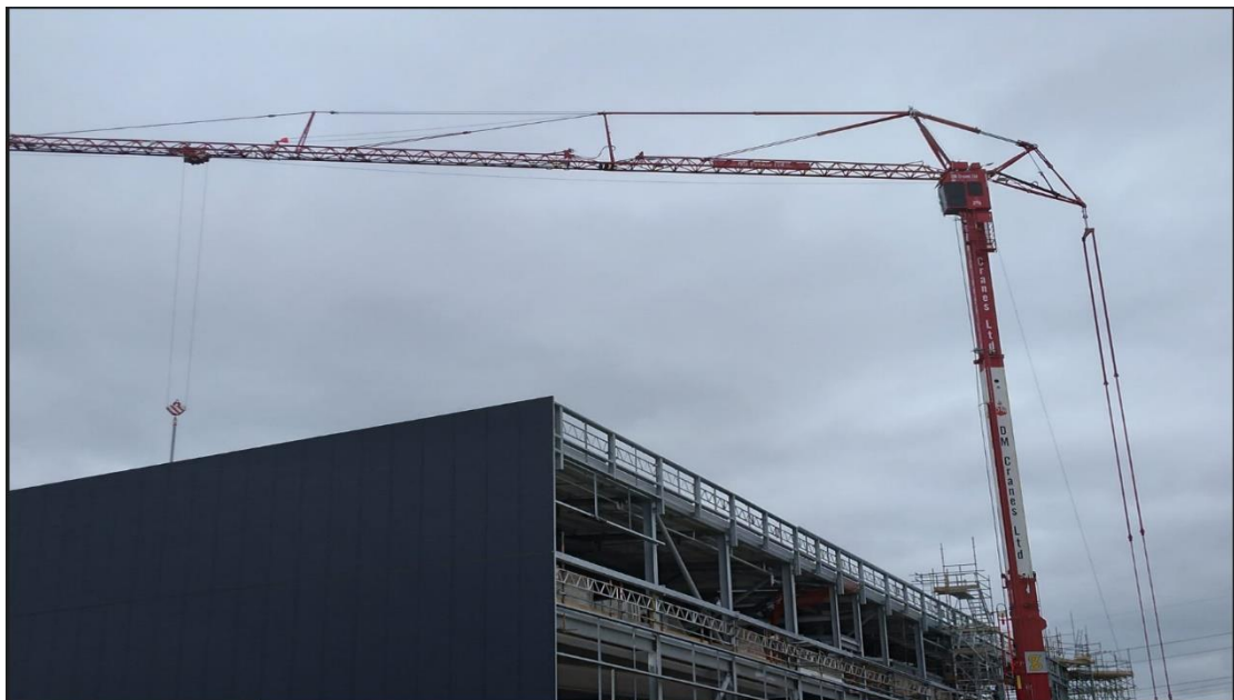
Electric tower crane at the RRF
