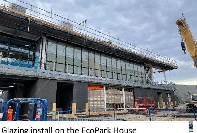
Glazing install on the EcoPark House
