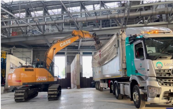
LEL Trialling Loading Operations on Tipping Apron
