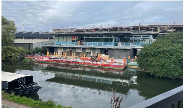
EcoPark House view from the River Lee Navigation
