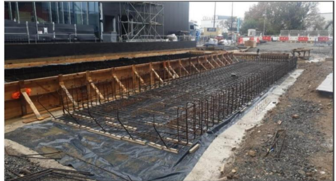
Rebar installation progress for 2nd Southern Weighbridge base
