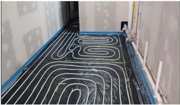
EPH G/F Underfloor Heating
