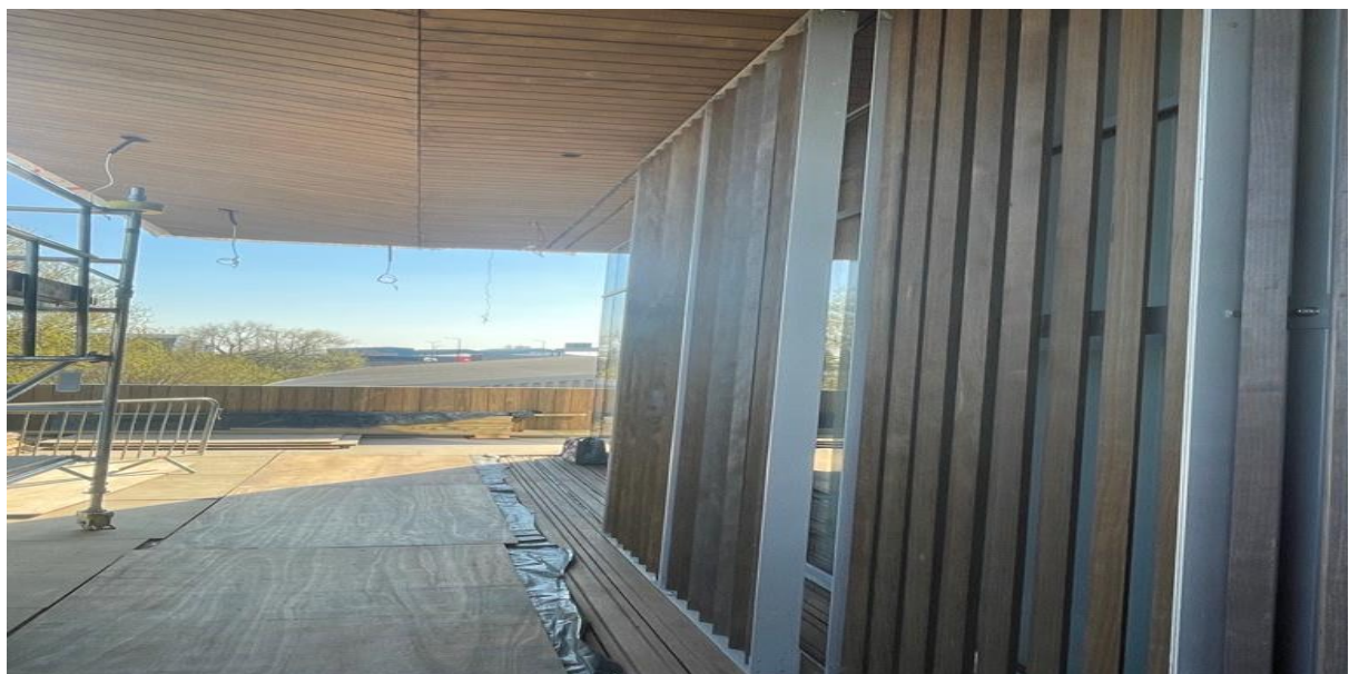
EcoPark House soffit and shutters installation
