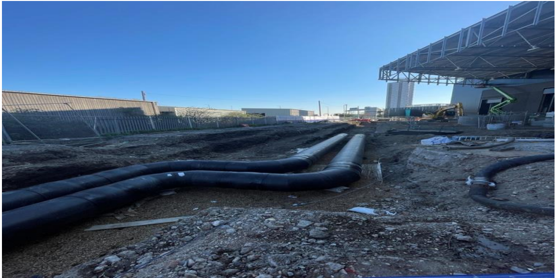
District heating pipe installation
