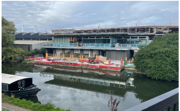
EcoPark House view from the River Lee Navigation
