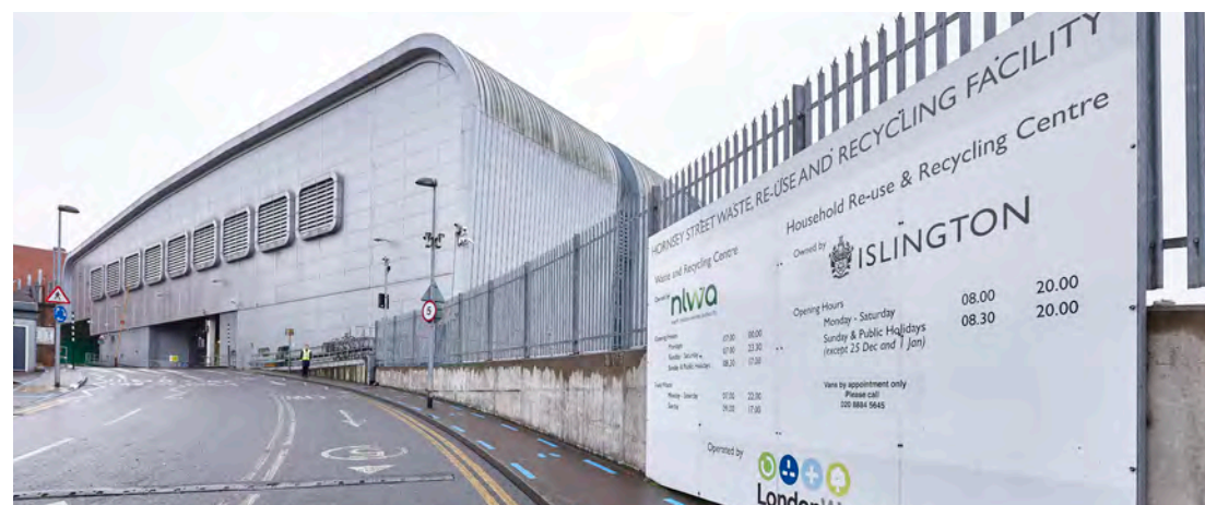
Hornsey Street reuse and recycling centre
