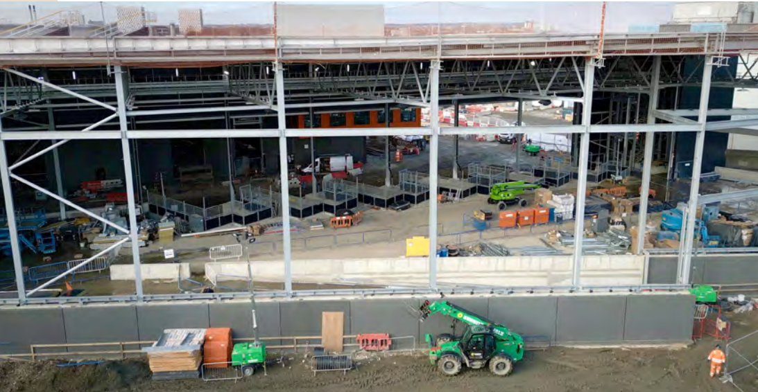
Reuse and recycling centre under construction
