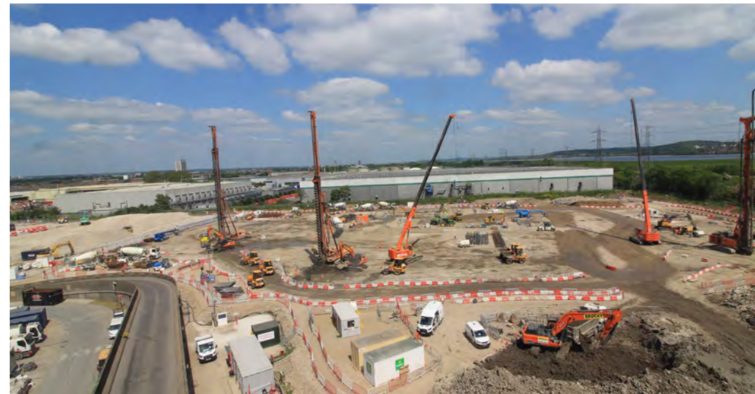
View of the eastern section of the ERF site under construction
