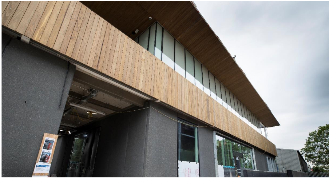
Western Elevation Timber Balustrades
