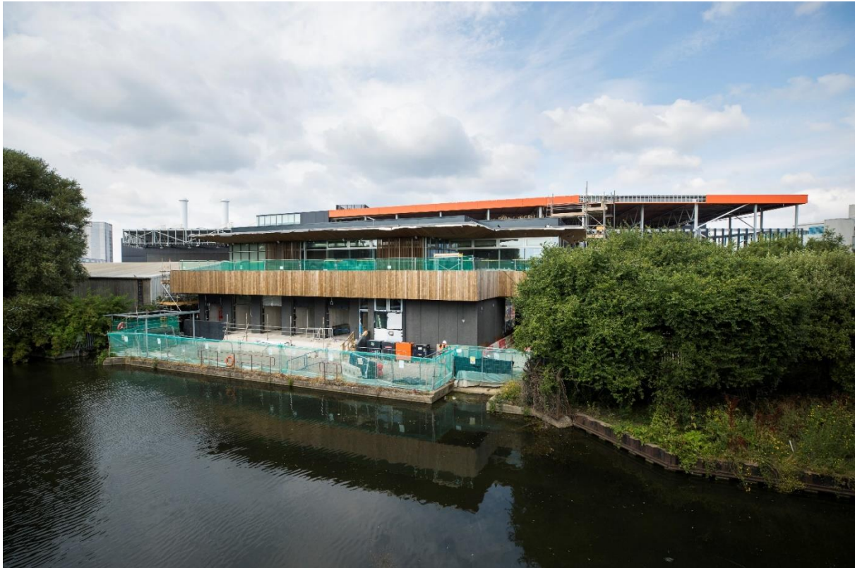
EcoPark House view from the River Lee Navigation
