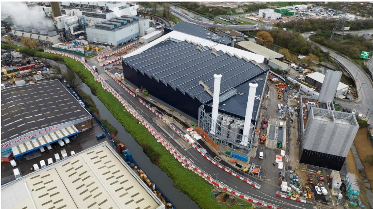
Aerial view of the RRF
