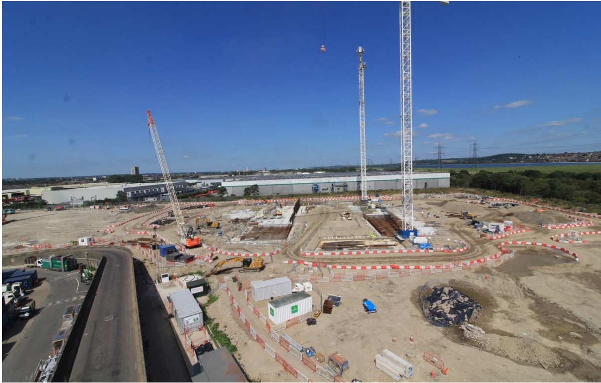
ERF construction site looking northwards
