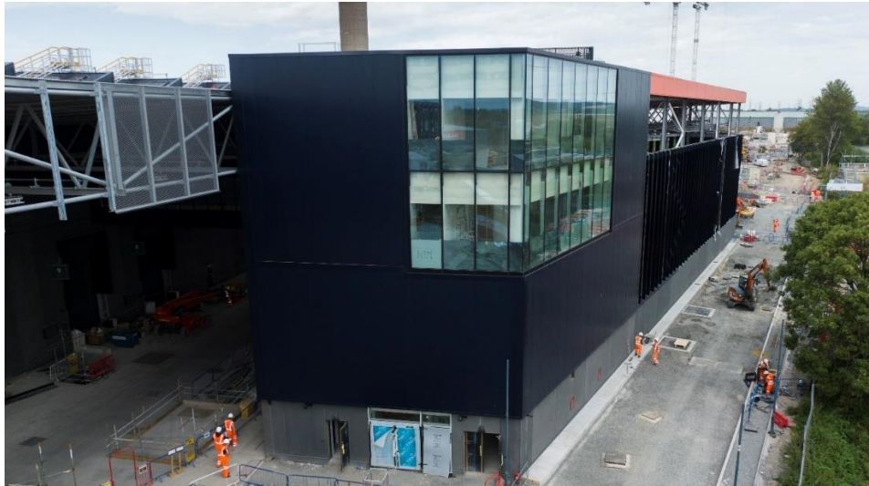
Figure 7: Eastern Access ramp
