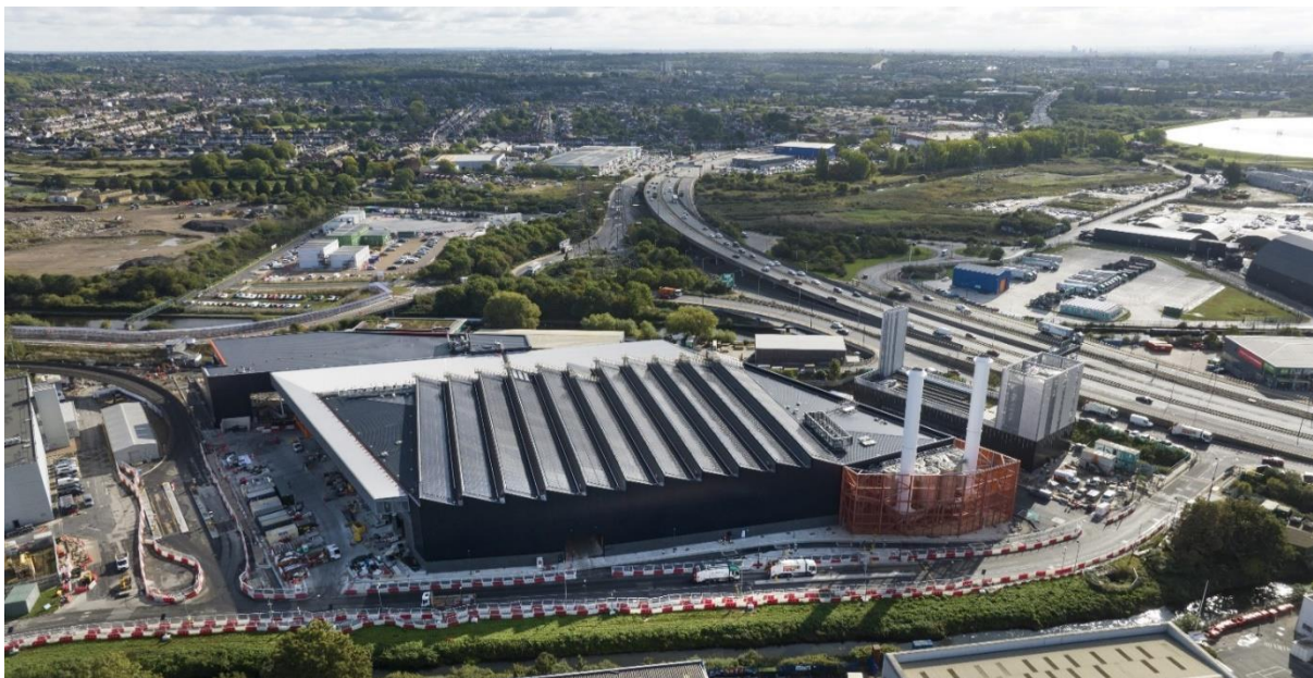
Figure 4: Aerial view of the RRF
