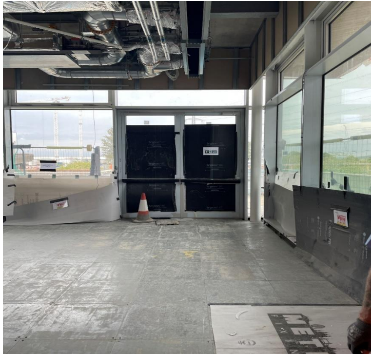
Figure 8: Exhibition Hall – civil elements installed
