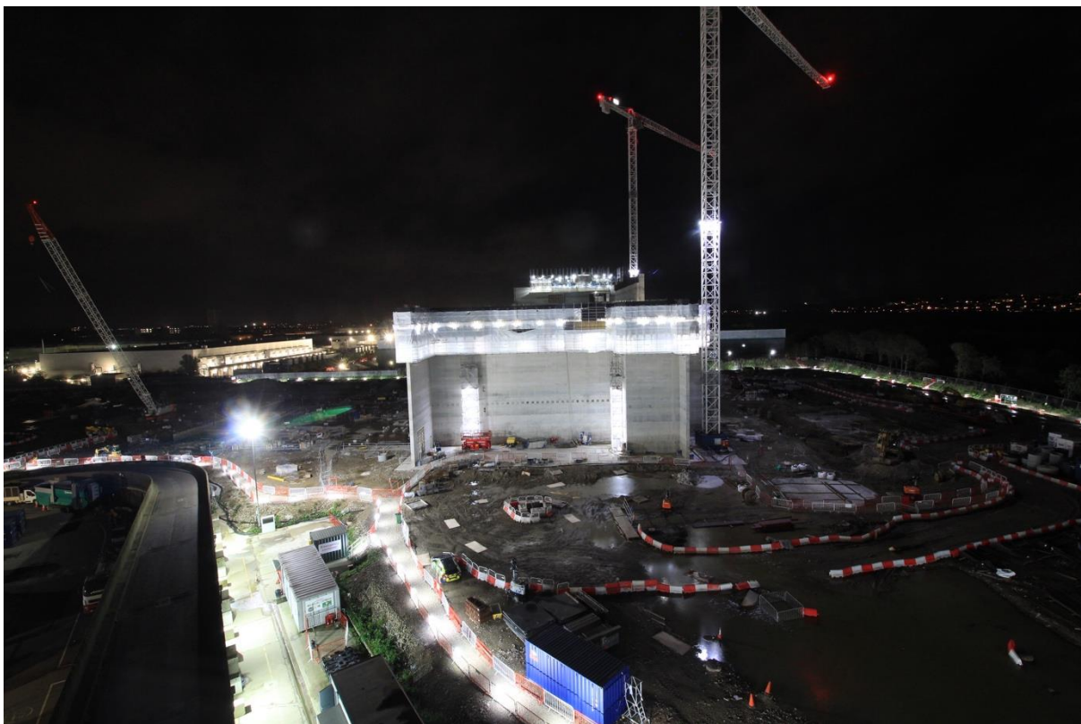
Figure 4: Completion of the Northern section of the bunker walls following four weeks 24/7 operations
