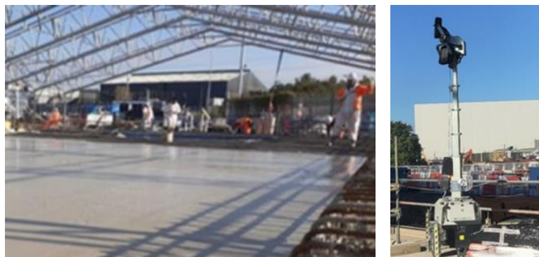
Figure 3: The ultra-low carbon cement-free concrete and an example of zero emission plant
