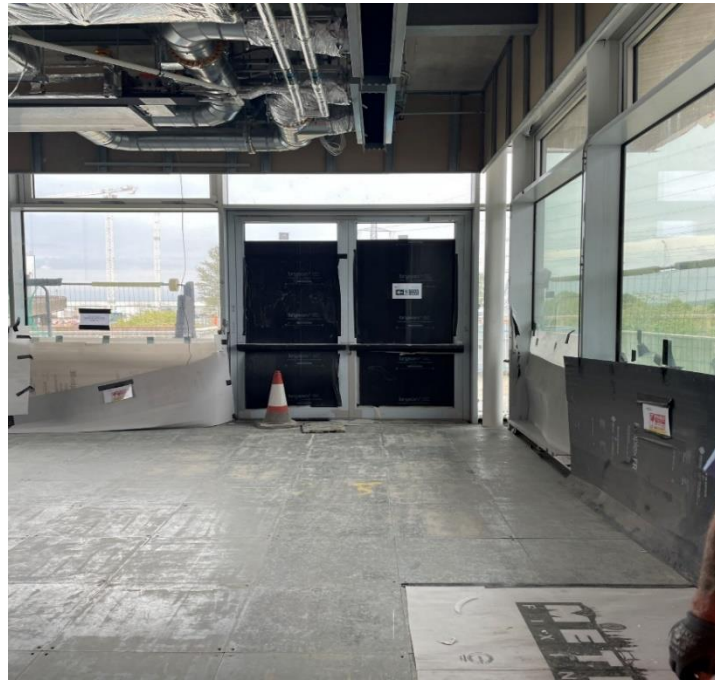
Figure 9: Exhibition Hall – civil elements installed
