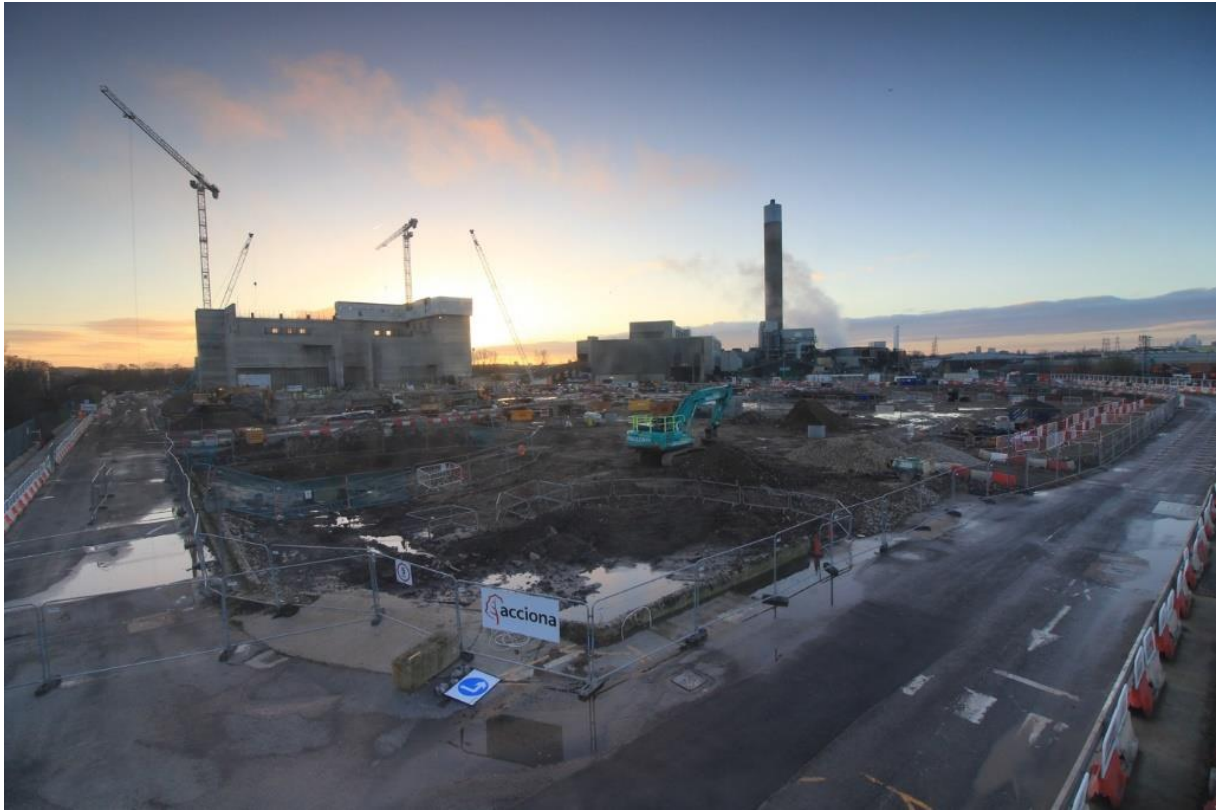
Figure 1: Completion of the bunker walls following 10 weeks of 24/7 operations
