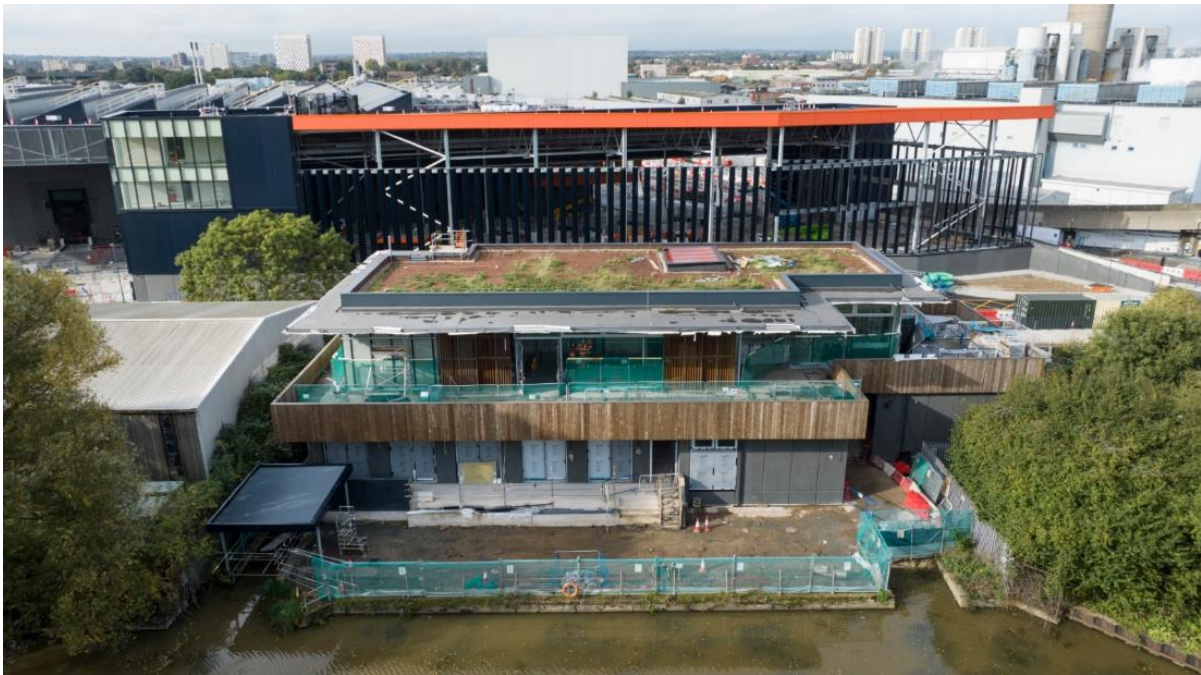
Figure 4: EcoPark House – canopy and decking – view from east
