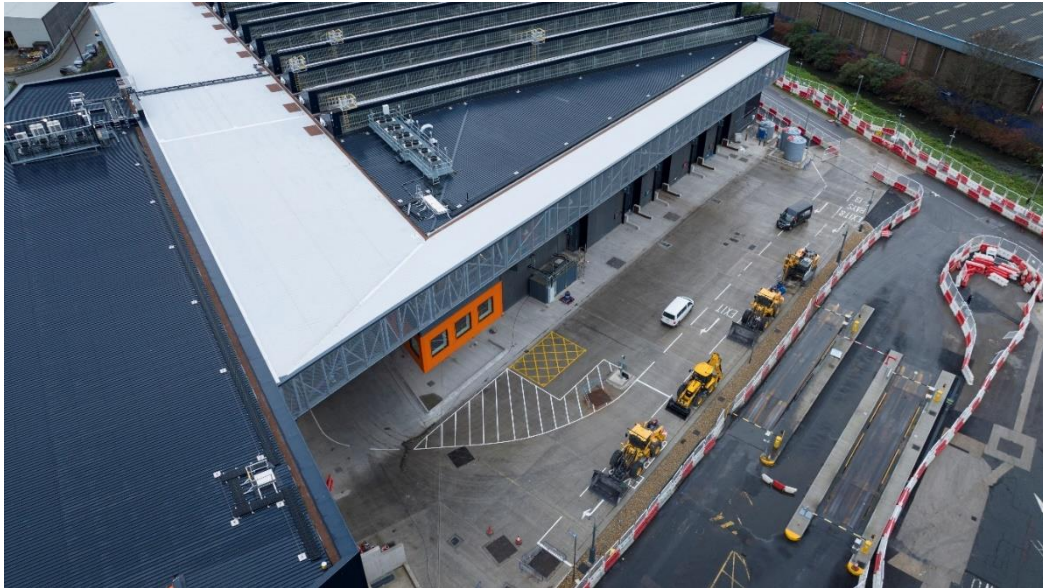
Figure 5: Northern Tipping Apron cleared in preparation for testing with waste
