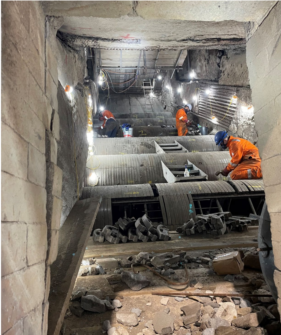
Figure 1: Planned outage works inside boiler 5, refurbishing of the roller grates
