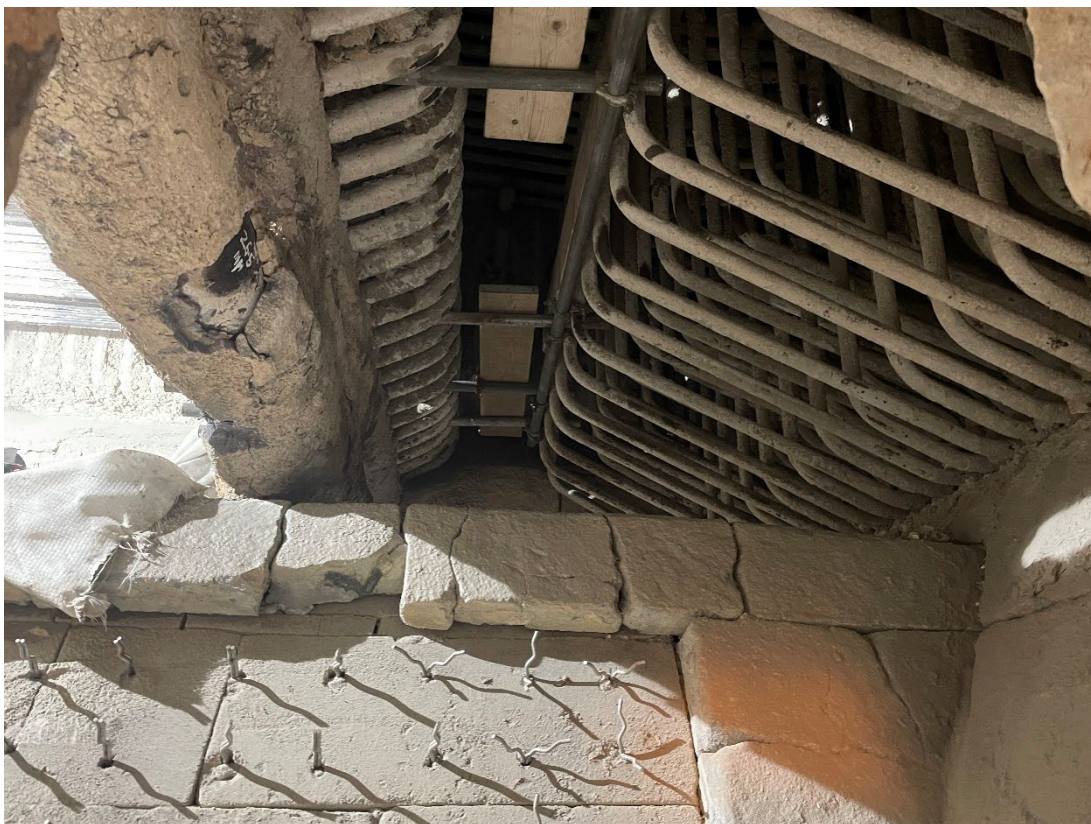
Figure 2: Steam tubes inside a boiler. Fixing some tube leaks requires Oxy-acetylene cutting and removal of healthy pipes to access the fault
