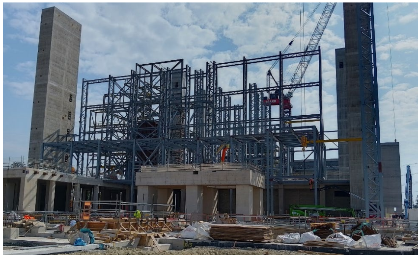
Figure 1: Turbine wall steelwork with turbine table in foreground
