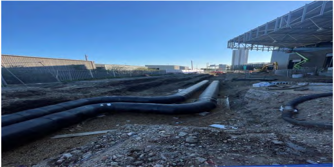
District heating pipe installation
