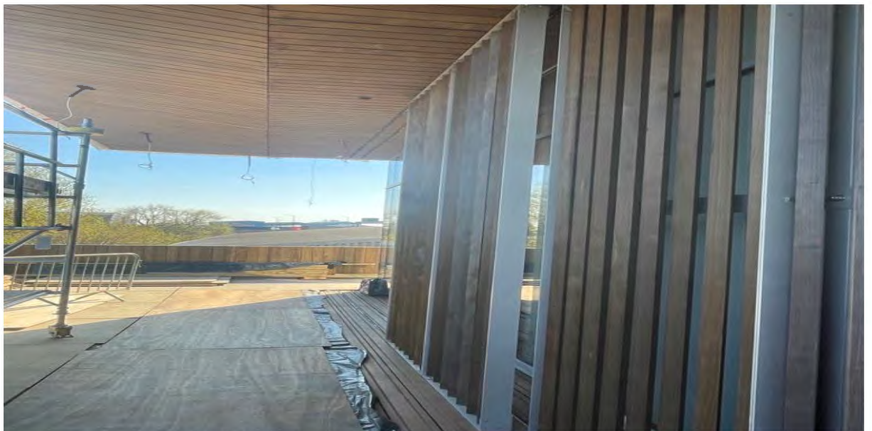
EcoPark House soffit and shutters installation
