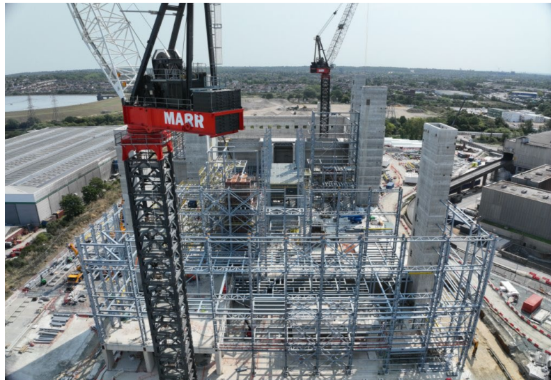
Figure 2: Turbine wall steelwork
