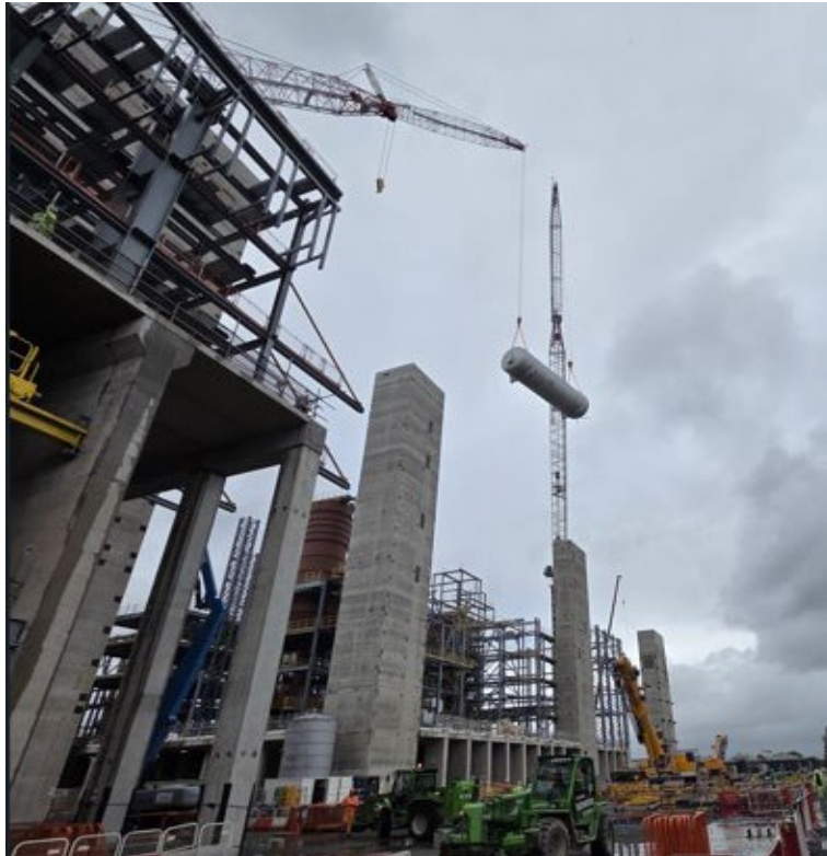
Figure 1: Boiler feed water tank installation
