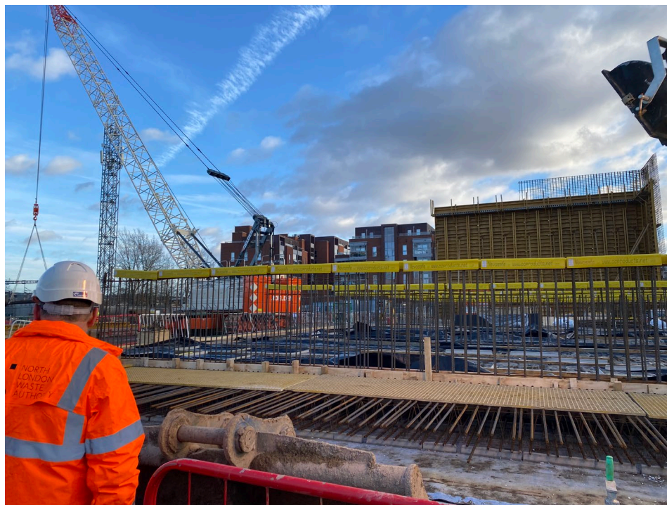
Figure 1: Site visit Geron Way 7th January 2026 showing steelwork for bays in place on one side of tipping hall
