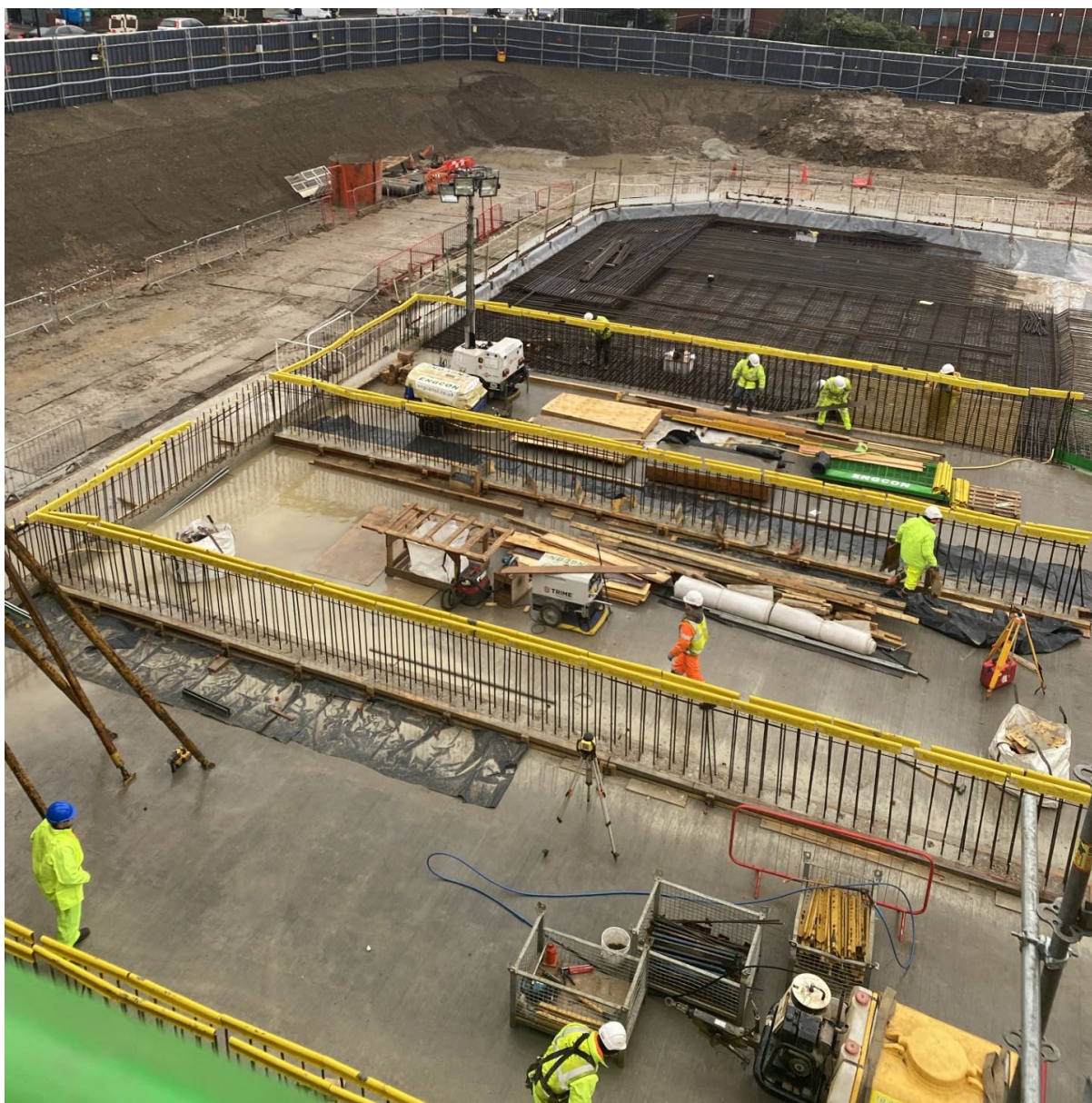
Figure 3: Site visit Geron Way 27th January concrete slab for bays now in place, preparing for pour of bay walls
