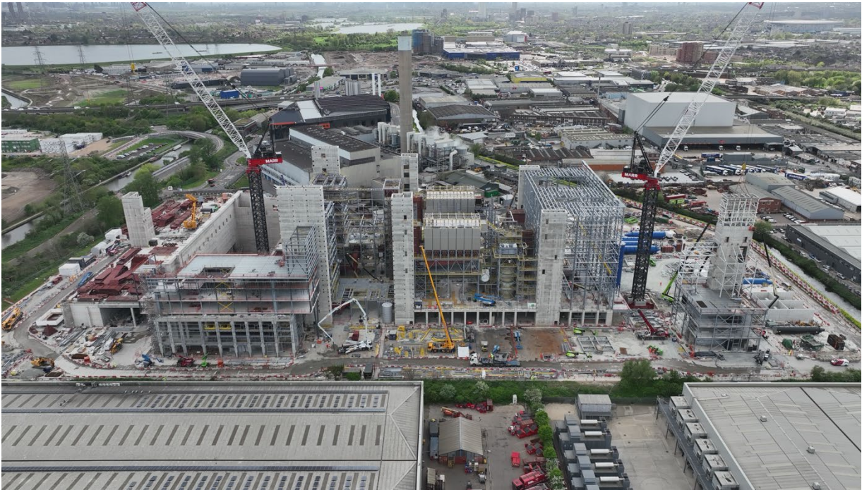
Aerial view of ERF construction progress as of April 2026
