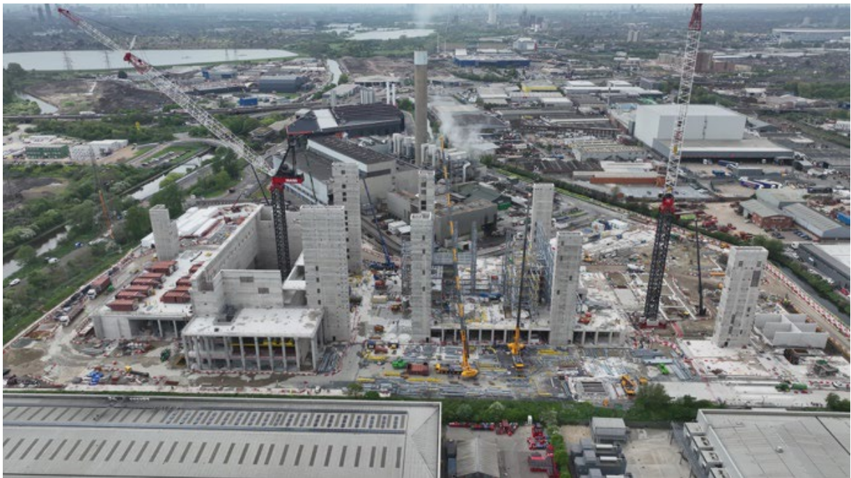
Aerial view of ERF construction progress as of April 2025
