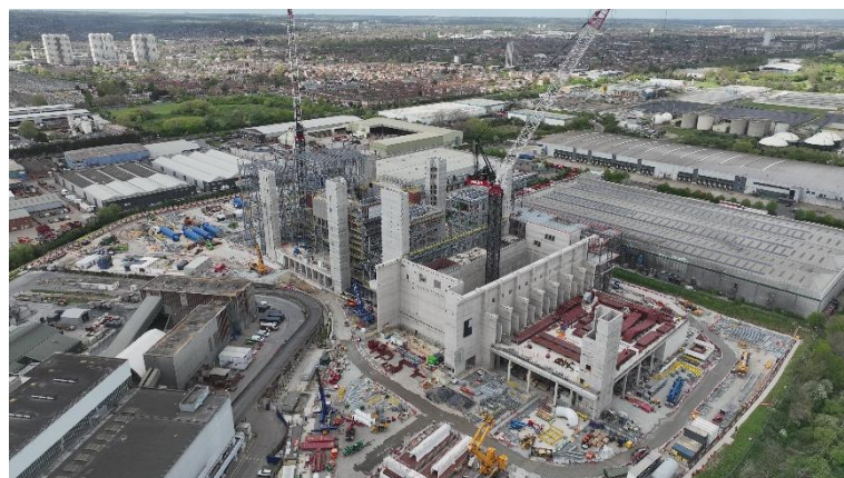
Construction of the ERF as at April 2026.
