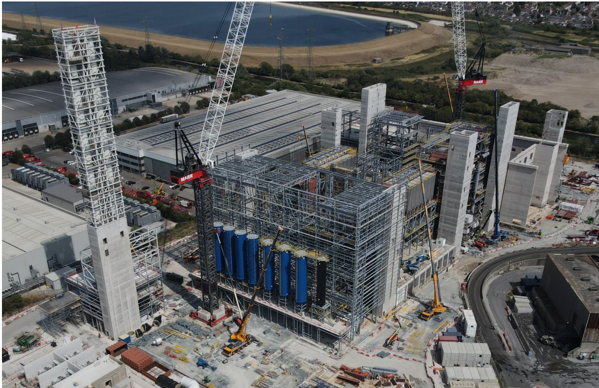
Figure 3: Silos (blue) in place, and stack progress July 2026
