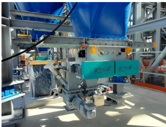
Figure 5: Silo valves and feeders, right waste hoppers for boilers
