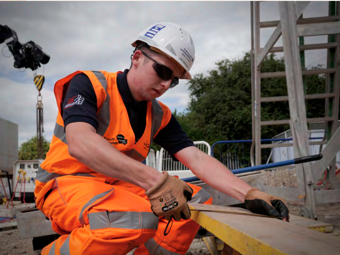
One of our many apprentices on site
