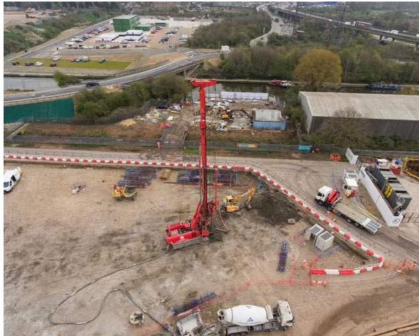
Image 1: Piling works being undertaken on EcoPark South, North London Heat and Power Project
