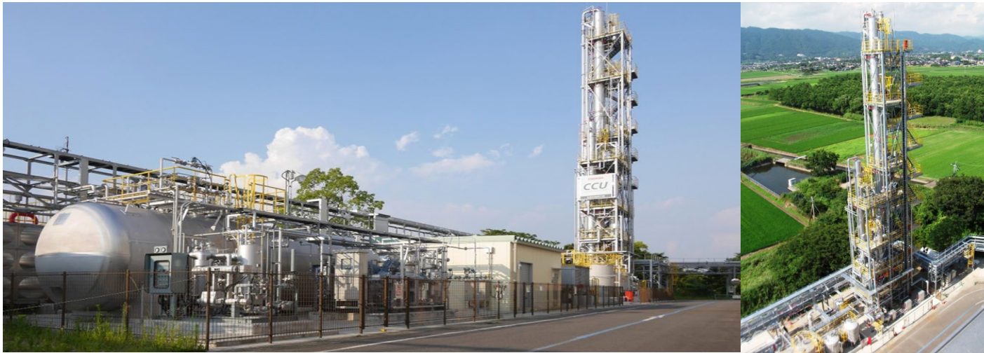
Figure 22: Toshiba Saga City EfW facility
