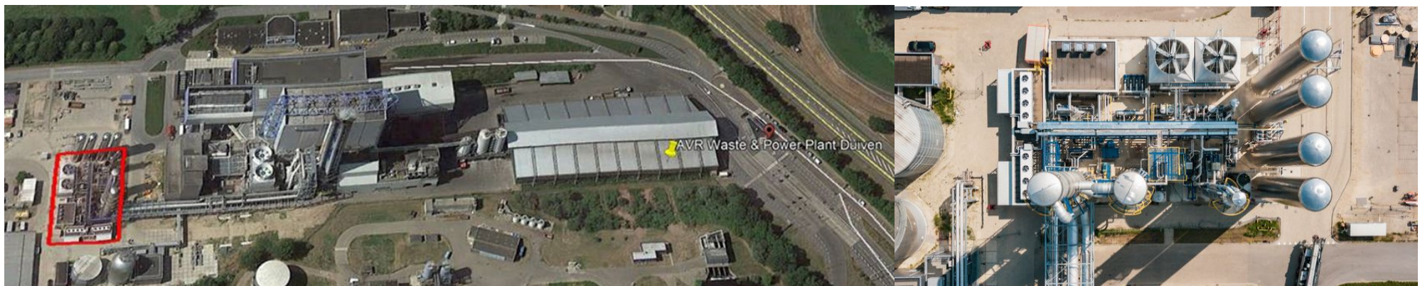
Figure 20: AVR Duiven CCUS facility (right image: overview of EfW facility with outline of carbon capture plant, left image: aerial view of carbon capture plant)
