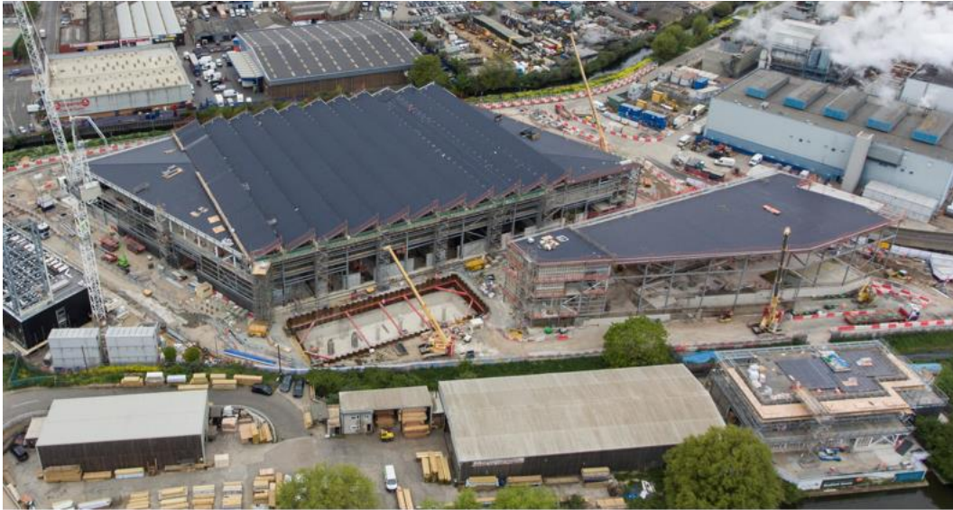
Aerial view of the RRF and RRC under construction with EcoPark House in the right foreground
