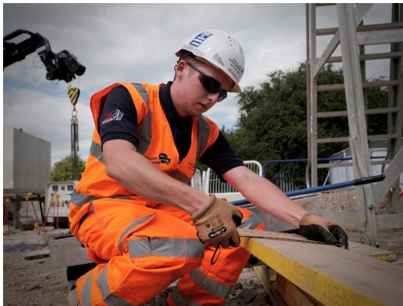
One of our many apprentices on site
