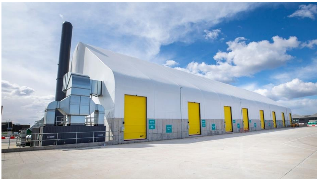
External view of the completed Temporary Bulky Waste Recycling Facility
