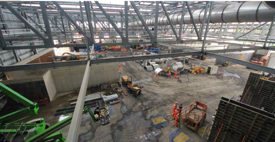
Internal view of the Resource Recovery Facility under construction
