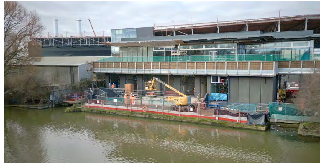
EcoPark House under construction
