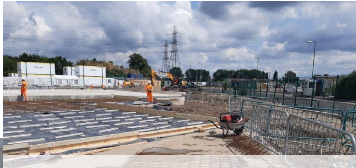
Image 2. Construction work on the temporary Transport Yard
